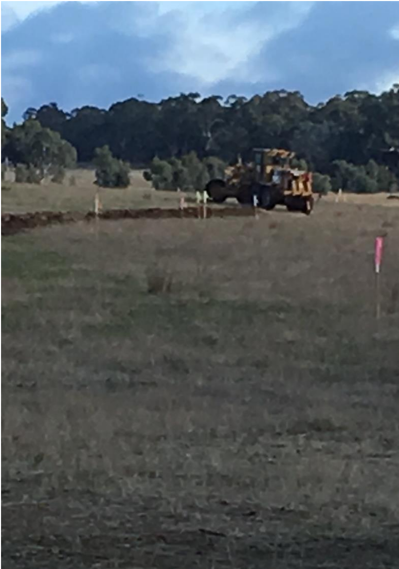
Figure 2 Start of Site Compound Works
