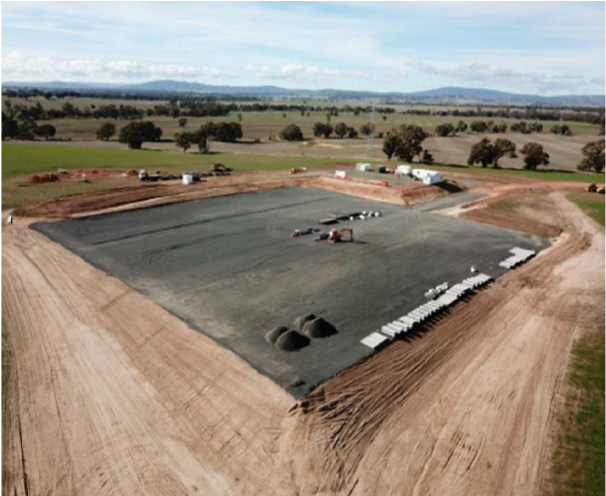
Figure 3 Terminal Station Pad Benching Construction
